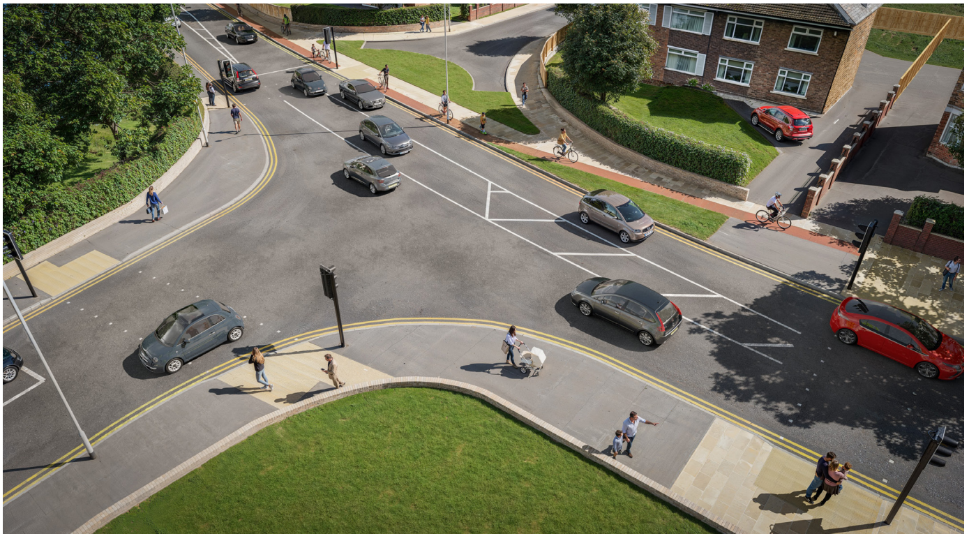
Indicative image showing three arm solution and new public realm, including shared pedestrian/cycle route
