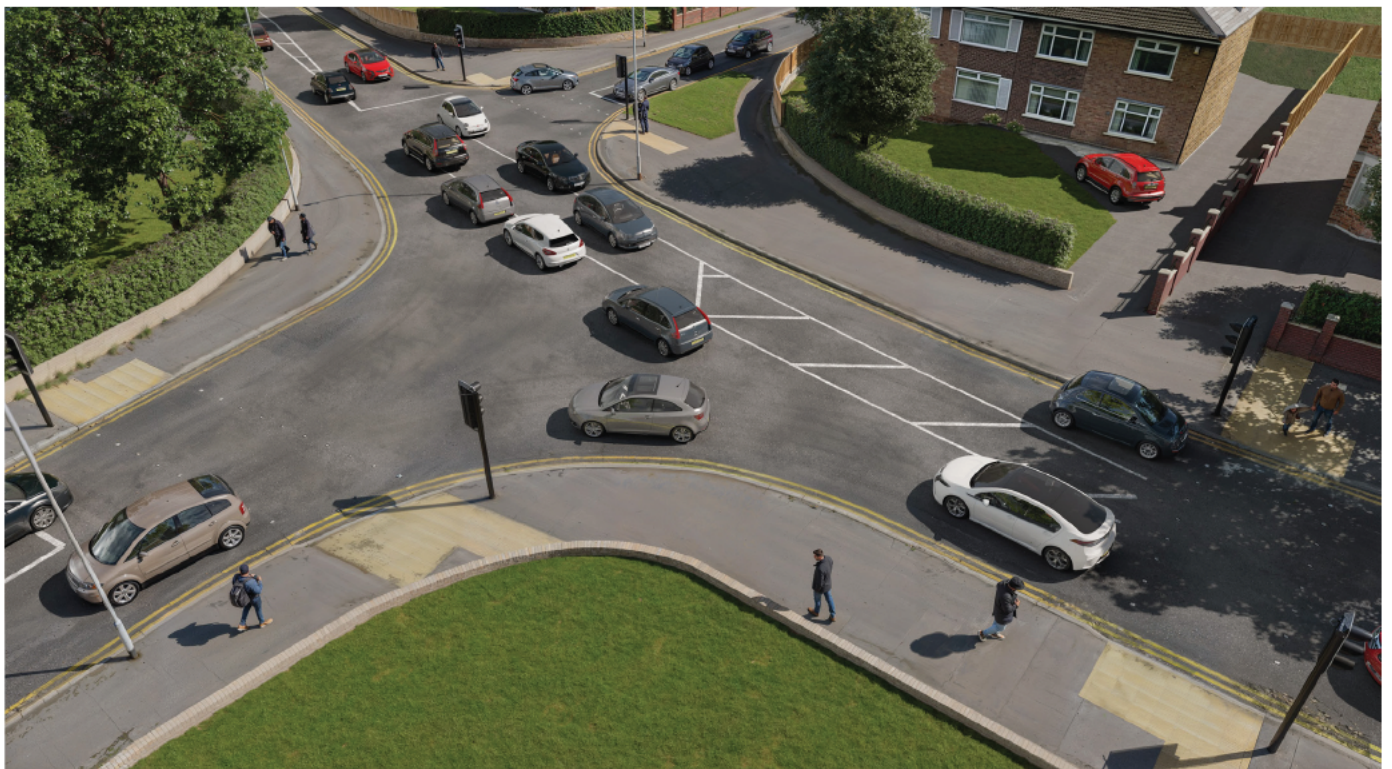
Indicative image showing four arm solution, including queuing for eastbound traffic turning right into Thackeray Grove
